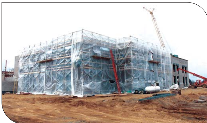
Figure 1. Masonry construction can proceed through winter months if an effective cold weather construction program is adopted. (IMG12504)
