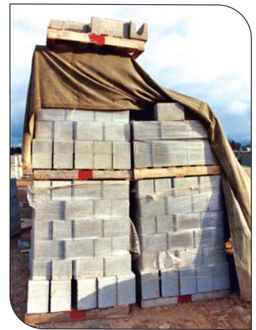
Figure 2. Masonry materials stored at the project need to be protected from rain, snow, and ice. (IMG12505)
